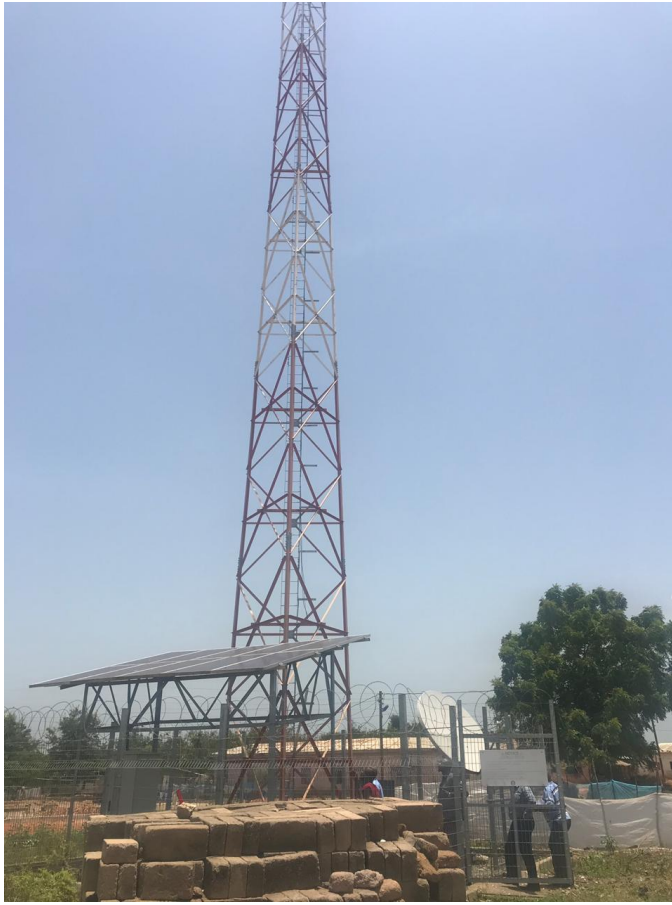
Figure 8 GIFEC RTP in Adidome, Volta Region
